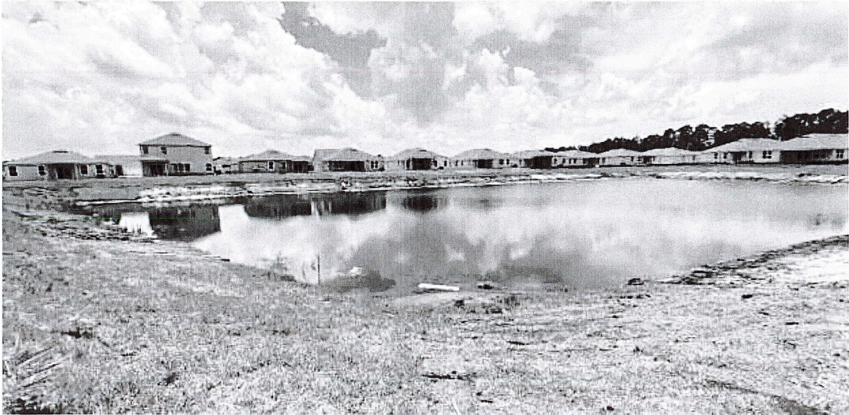
Lake #15. 698 Navarez Ave. 1.6 acres 1100' shoreline. Water level low. Minimal aquatic weed growth present. Access for truck and treatment boat will need to be provided unobstructed at 698 Navarez Ave
